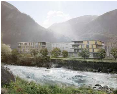
Stalon - Roveredo, Switzerland / 2017 Floor area 5860 smq
