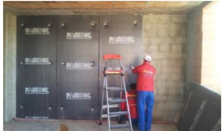
Laying insulating wall
