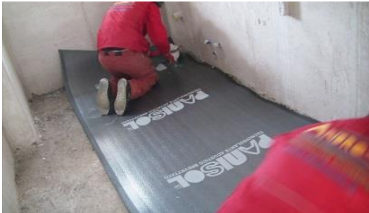
Laying floor insulation
