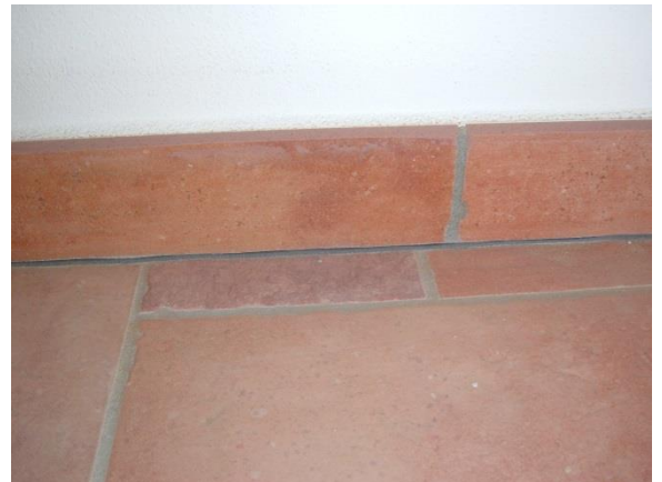
SKIRTING BOARDS IN CERAMIC FILLING SILICONIZED HORIZONTAL CORRECT PROCESSING
