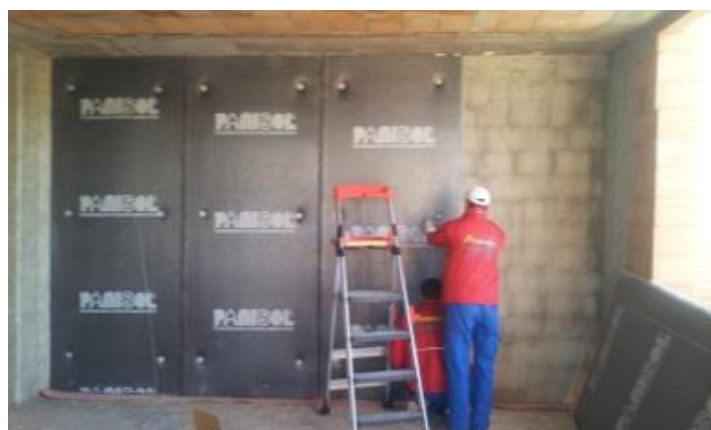
Laying insulating wall
