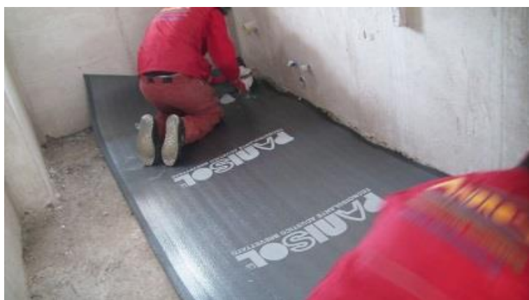
Laying insulating to treading
