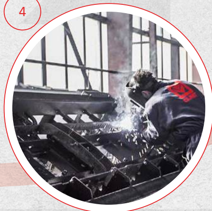
Supply, assembling works, start-up
