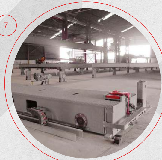
Components to provide pallet circulation
