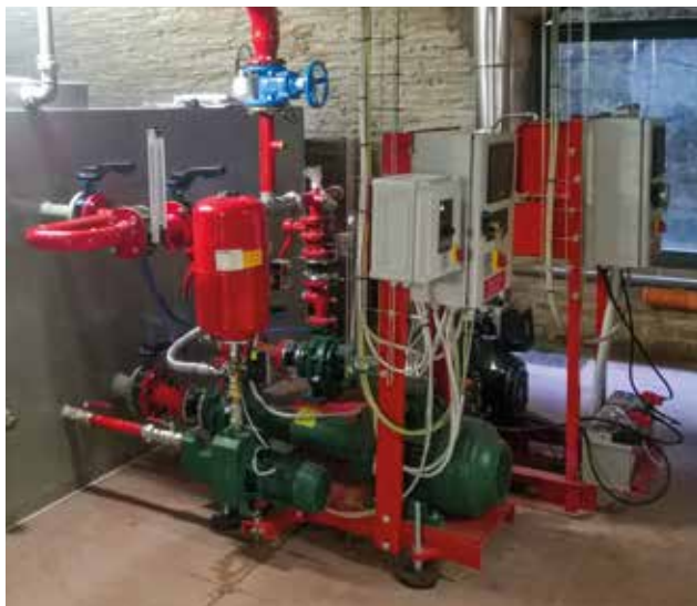
Plant constructed directly on site
