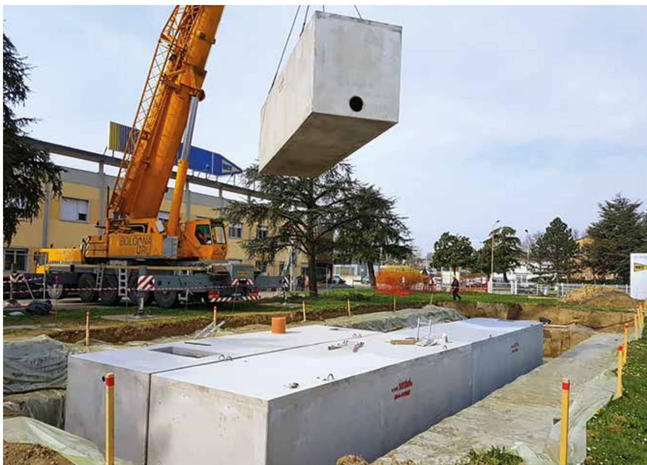
Underground reinforced concrete tank
