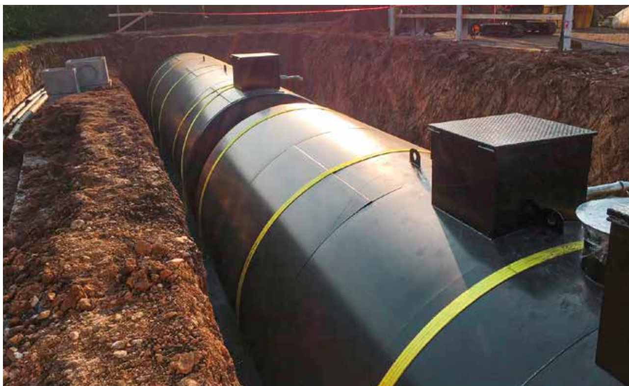
MF CI-TIC system with anchoring system
