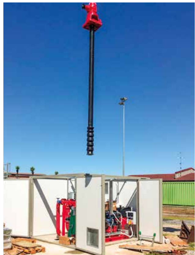
Shaft line installation detail
