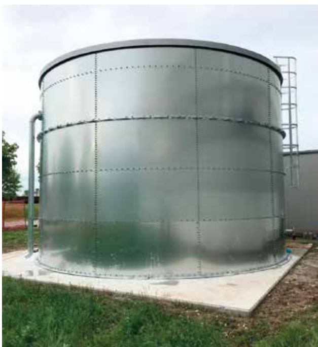
MF CO-TW 200 m³ + TBOX - Rail cargo terminal - Venice
