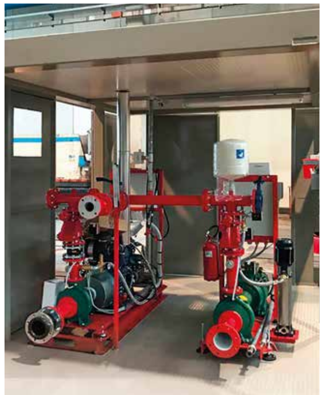
Fire pump room under construction
